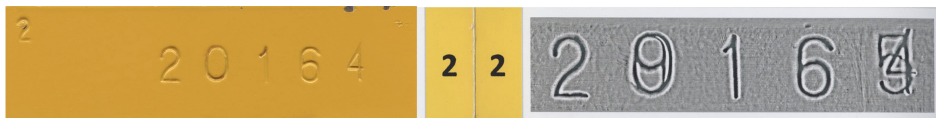
Filling symbols with tin (soldering)
